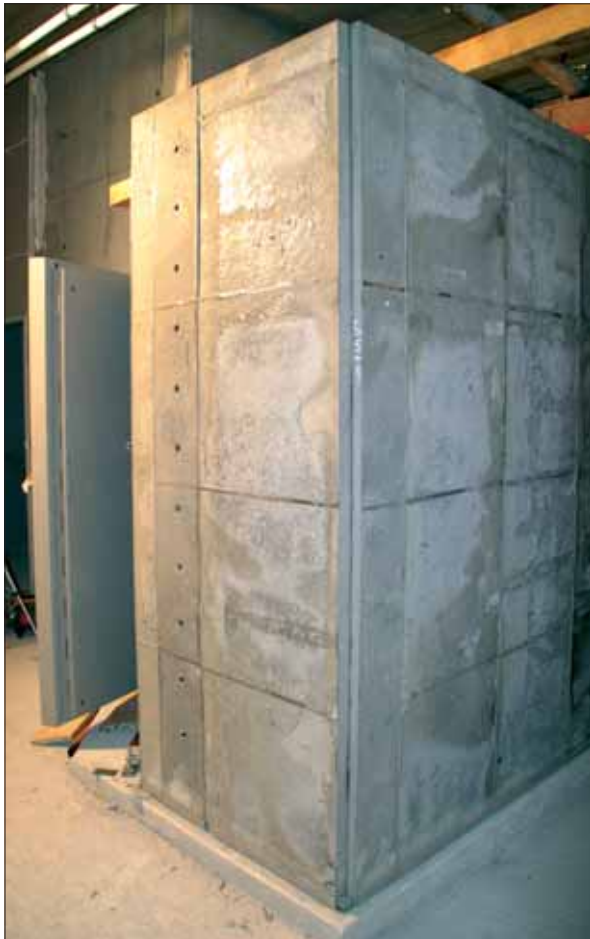
Elements of prefabricated vault EET 070 with vault door EWT 085
