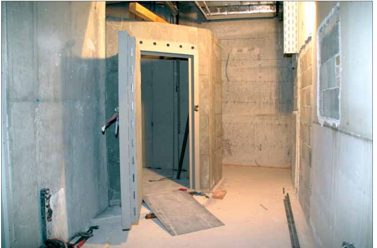
Elements of prefabricated vault EET 070 with vault door EWT 085
